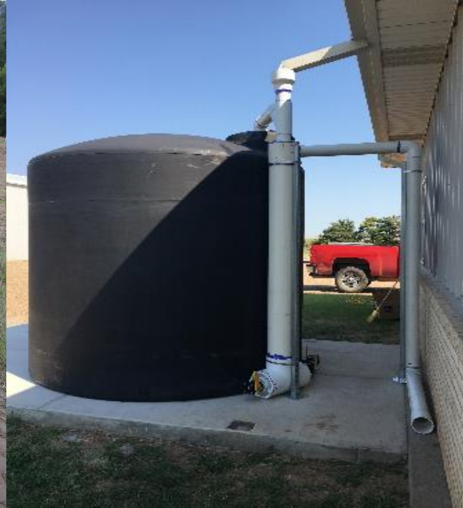
Irrigation Reservoir (Water Catchment)
